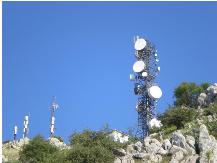
Figure 6-2: Steel lattice telecommunication tower
